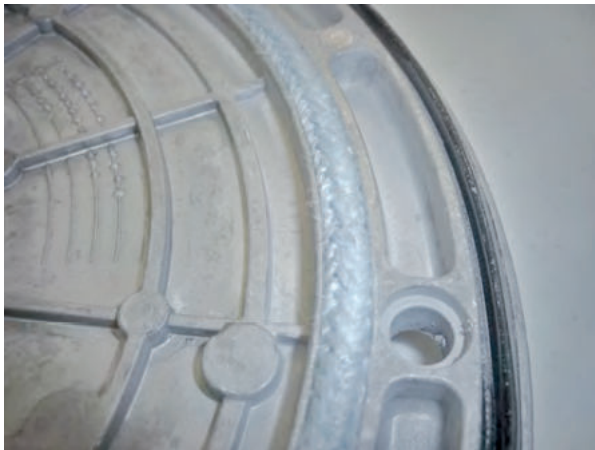
Rope gasket in good condition
